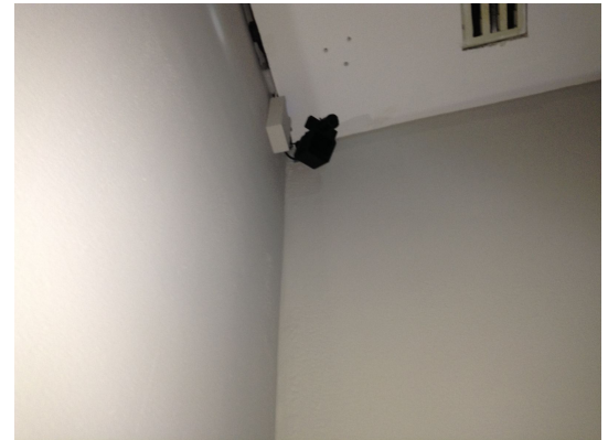
White box beside corner camera
