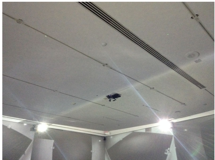
Ceiling cameras, IR illuminator, and USB extenders in the middle of the ceiling
