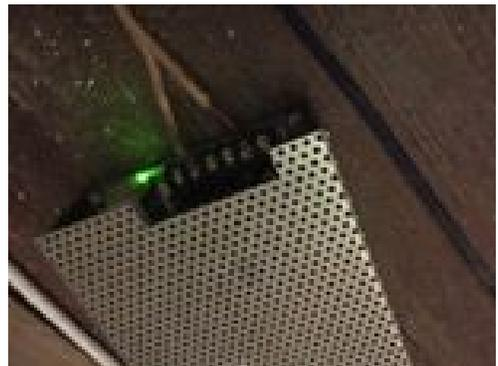
Next, connect the power cable to the power supplies behind the wall, on the side of the power supply with six terminals. The cable with the stripe connects to the 24V live (L) terminal, and the cable with no stripe connects to the 24V neutral (N) terminal.
