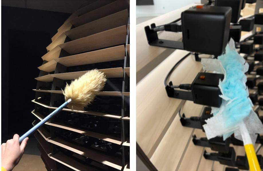
We recommend undusting the wood slats and metal structure with a microfiber cloth as the edge of the slats are very fragile so no pressure should be applied. Slightly dampen said microfiber cloth to remove marks and residues from the wood slats and speakers.
