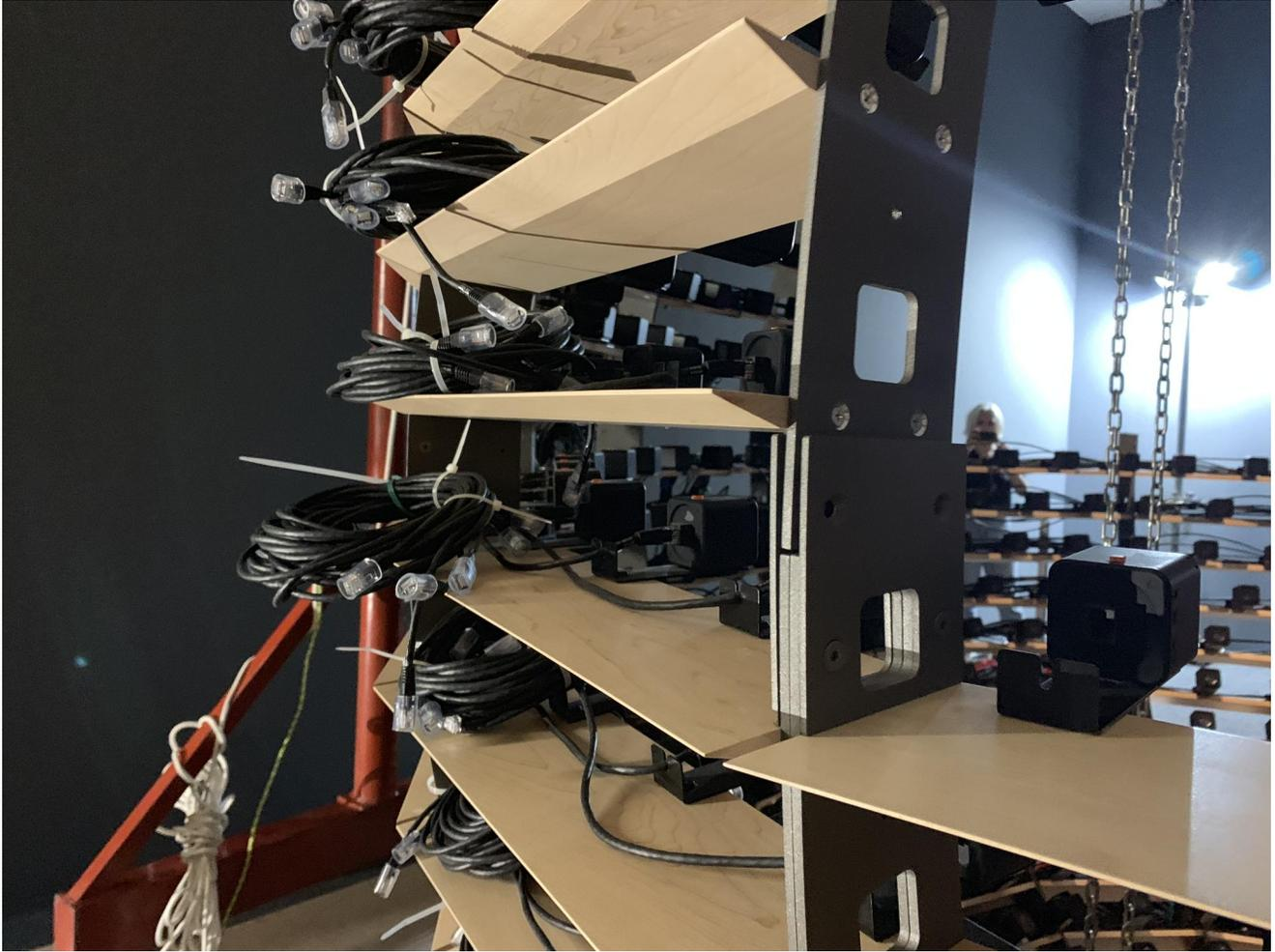
Install the other quarter containing cables and complete the top with the two front parts (without cables) last.
