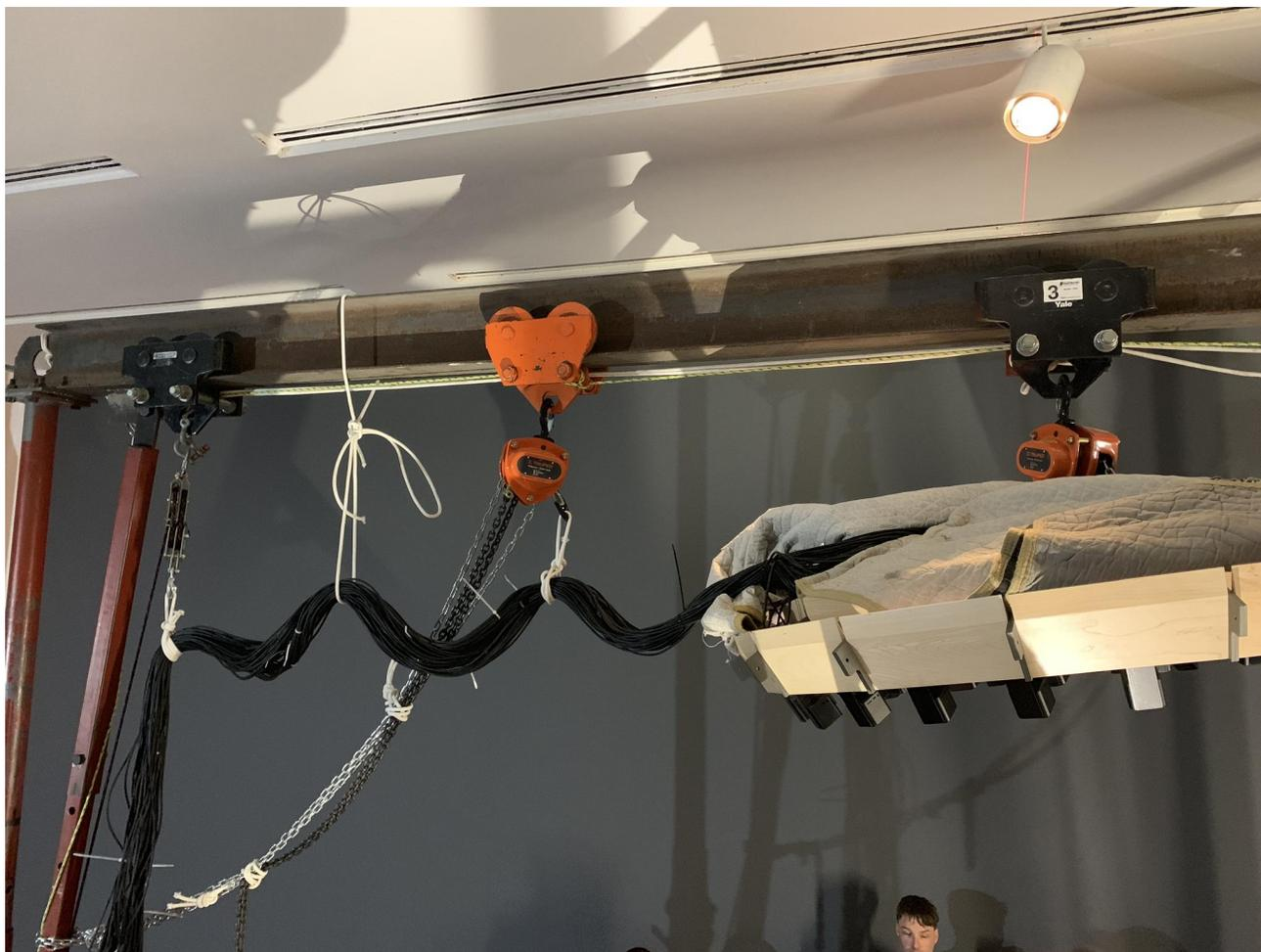
Have a person inside the sphere on a ladder that can come and receive the dome and make sure it fits within the brackets. Once it is in position, the person inside the sphere can insert screws loosely, and in the same fashion as for the other parts of the sphere, only tighten every screw once it is in place.
