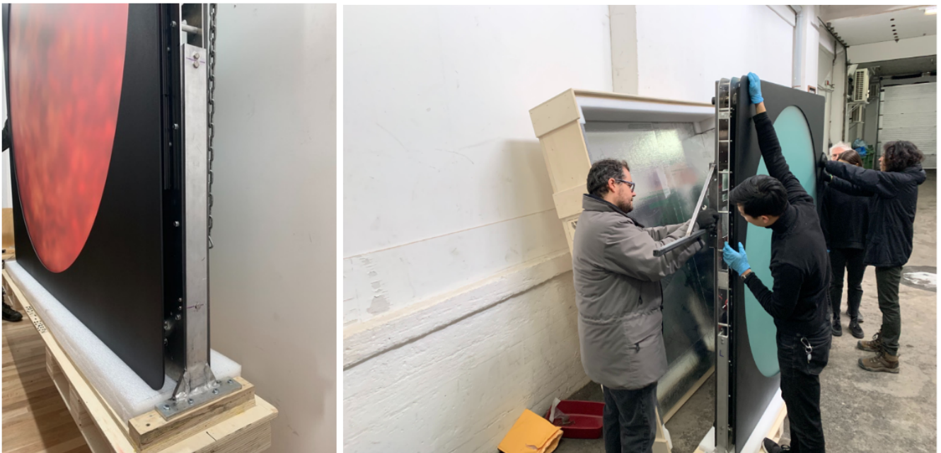
Brackets on base of crate keep the display securely in place during shipping and installing
