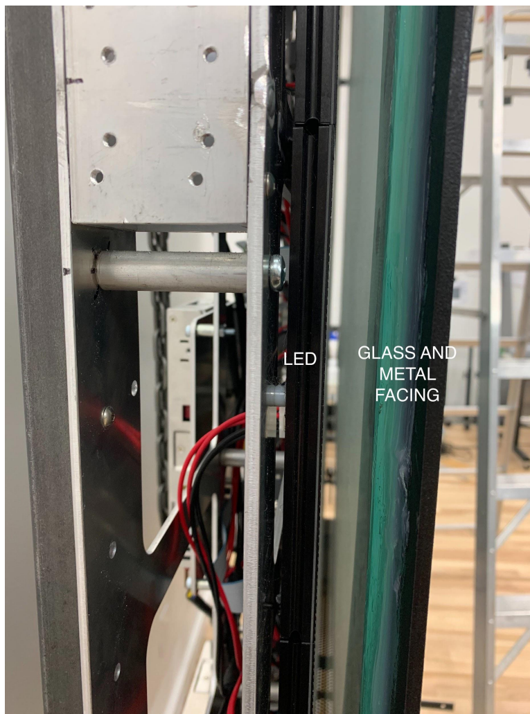
Side view of segments; gap between LED panels and glass and aluminum facing.
