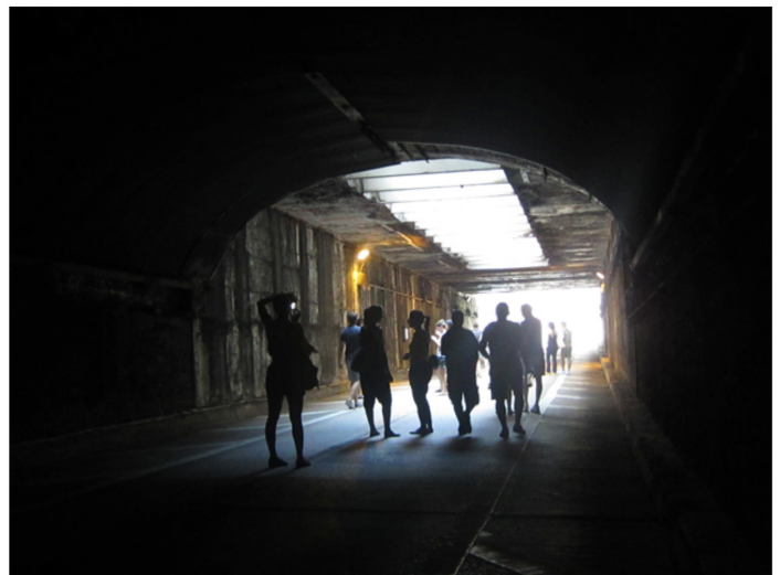
Exiting the Park Avenue Tunnel
